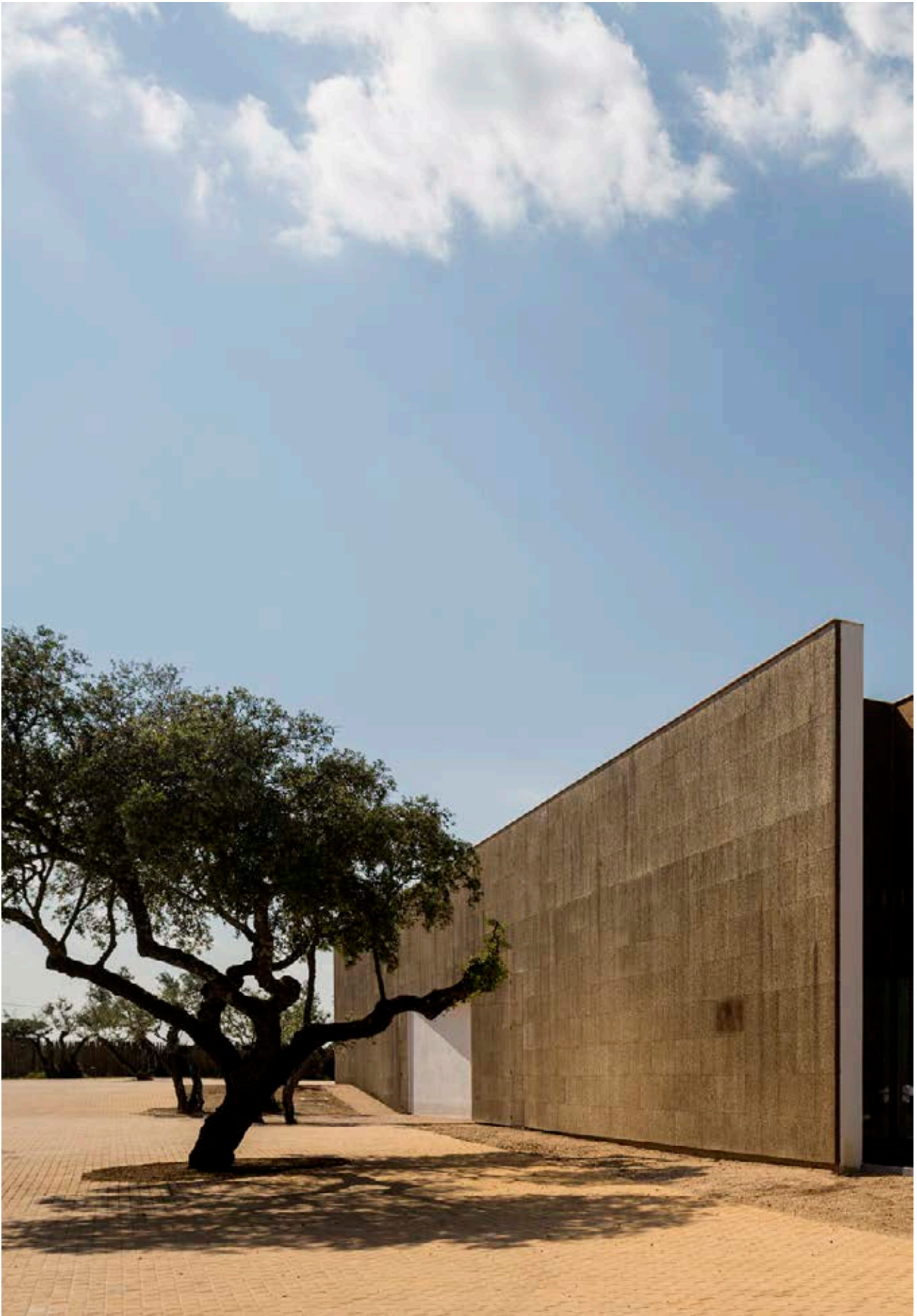
ECORKHOTEL, IN ÉVORA, PORTUGAL, WITH ITS FAÇADE COVERED WITH EXPANDED INSULATION CORKBOARD MANUFACTURED BY AMORIM ISOLAMENTOS
