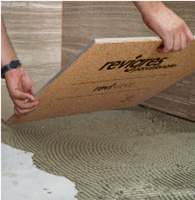
REVISILENT, AN INNOVATIVE FLOORING COMBINING A CERAMIC FLOOR TILE WITH A CORK UNDERLAYMENT
