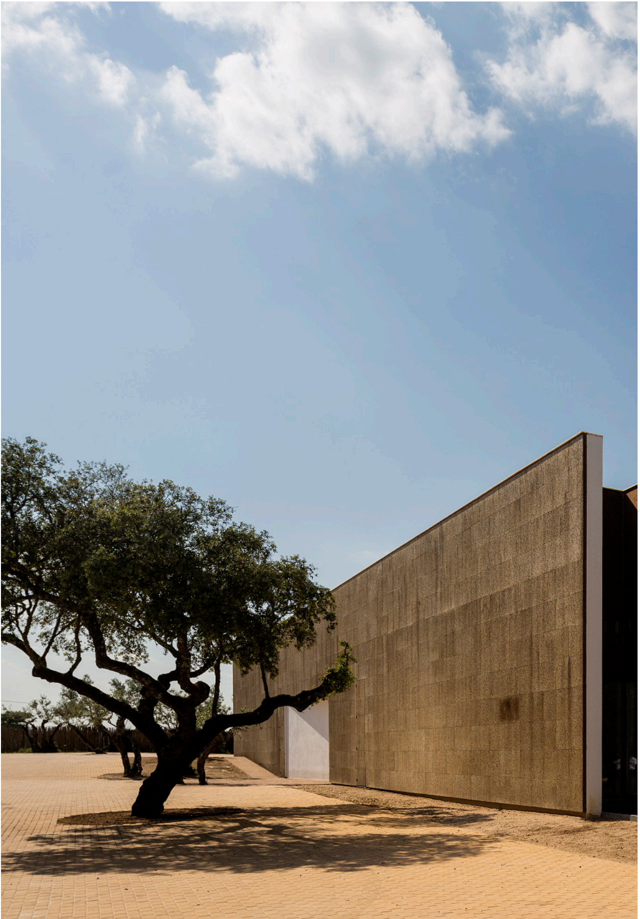
ECORKHOTEL, IN ÉVORA, PORTUGAL, WITH ITS FAÇADE COVERED WITH EXPANDED INSULATION CORKBOARD MANUFACTURED BY AMORIM ISOLAMENTOS
