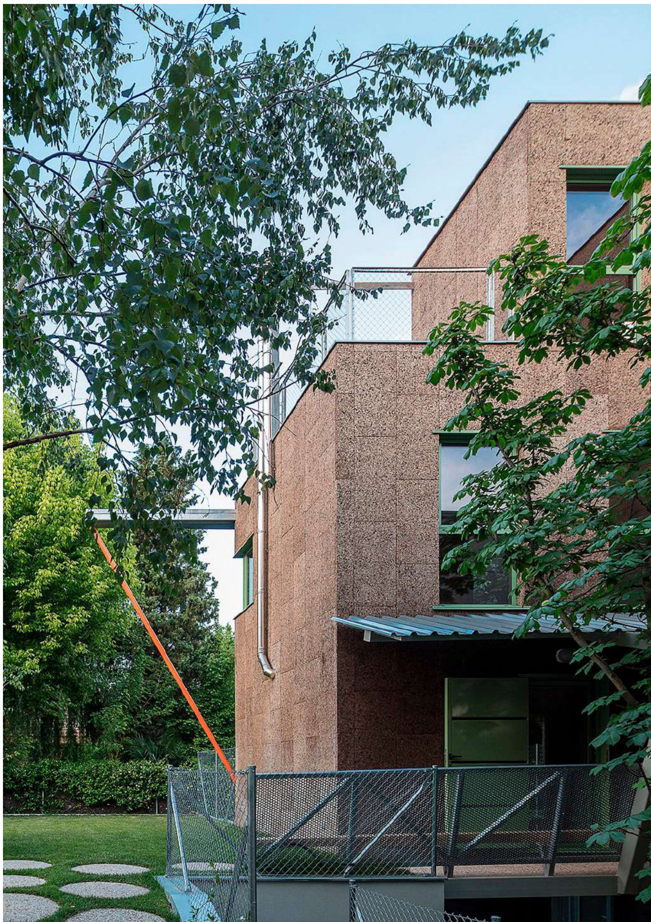
Designed by Spanish architects Teo Nuñez and Almudena Ribot, the "Casa Pádel" in Madrid seamlessly integrates a wooden structure with expanded cork cladding from Amorim Cork Insulation.
