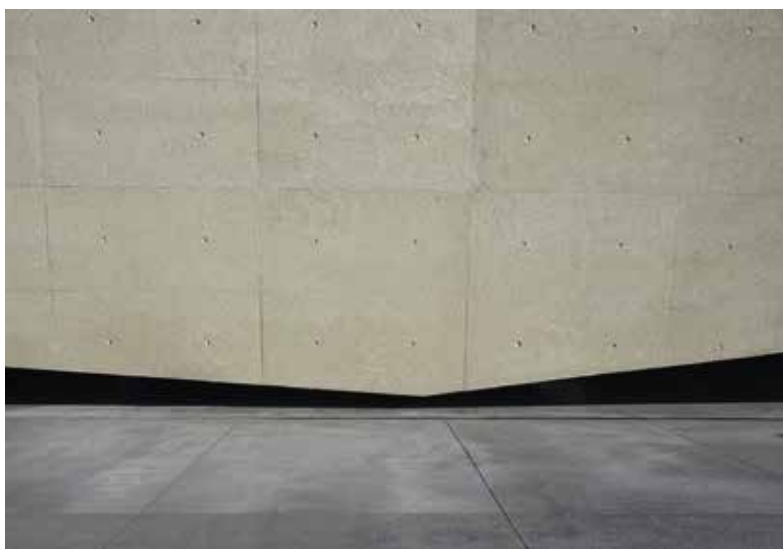
Lisbon Cruise Terminal that uses a type of light structural white concrete mixed with granulated cork.
