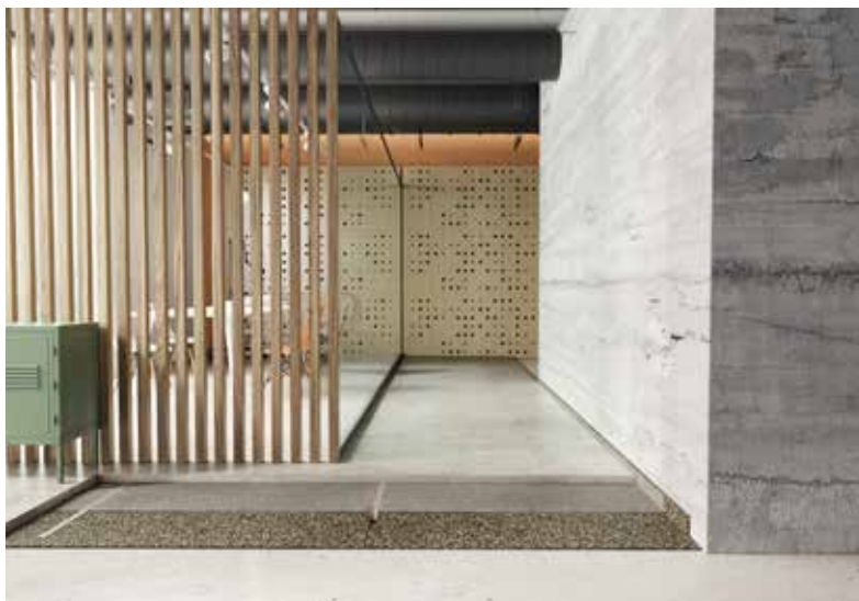
Amorim Cork Composites' underscreed, installed beneath the final floor, provides sound insulation.
