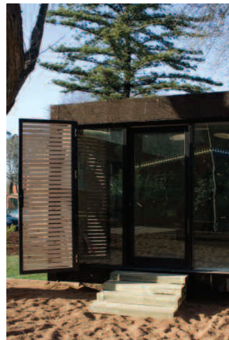
Amorim Isolamentos presented the Eco-cabin project, a new accommodation concept designed for ecological tourism, which has the novelty of being totally covered and insulated with cork.
