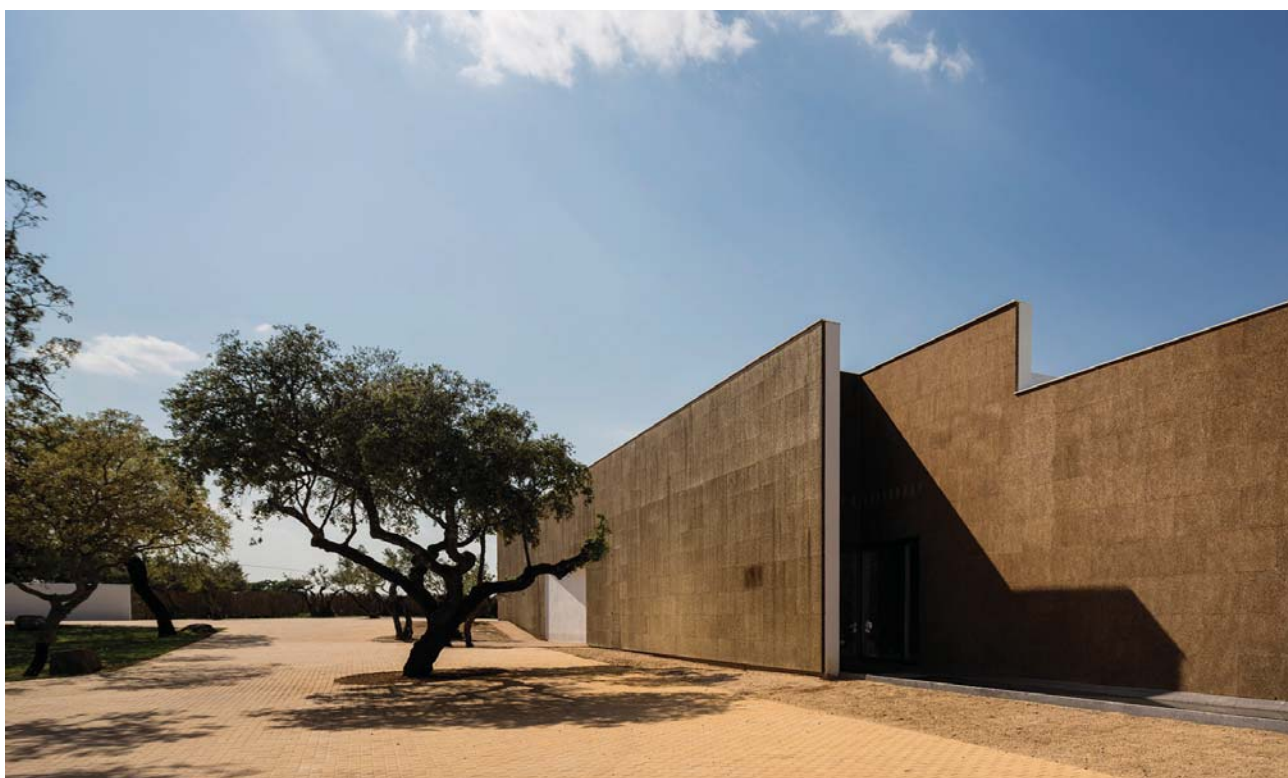
HOTEL COVERED WITH EXPANDED INSULATION CORKBOARD
