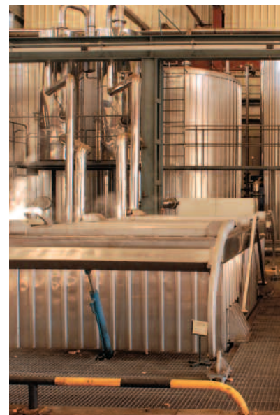
Cork boiling system. The revolutionary Convex system for boiling cork assures that water is constantly filtered thus enabling its reuse.
