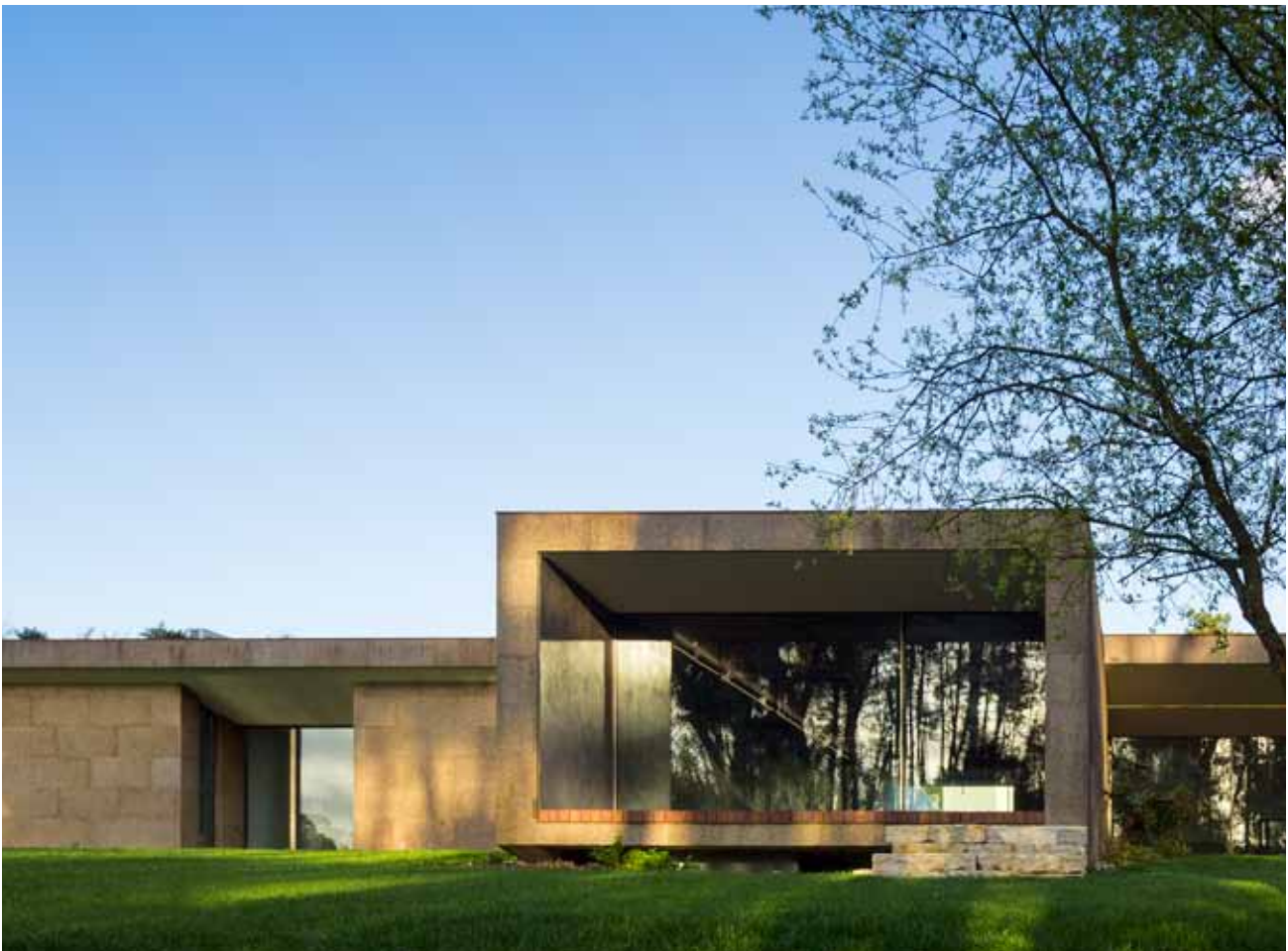
PRIVATE HOUSE COVERED WITH EXPANDED INSULATION CORKBOARD
