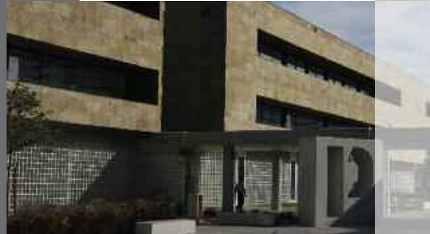
Pedro Arrupe College: the façade is covered with expanded cork agglomerate
