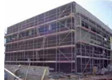
**Photograph 1 – Prepared façade / insulated with cork for placement of ETICS finishing**
