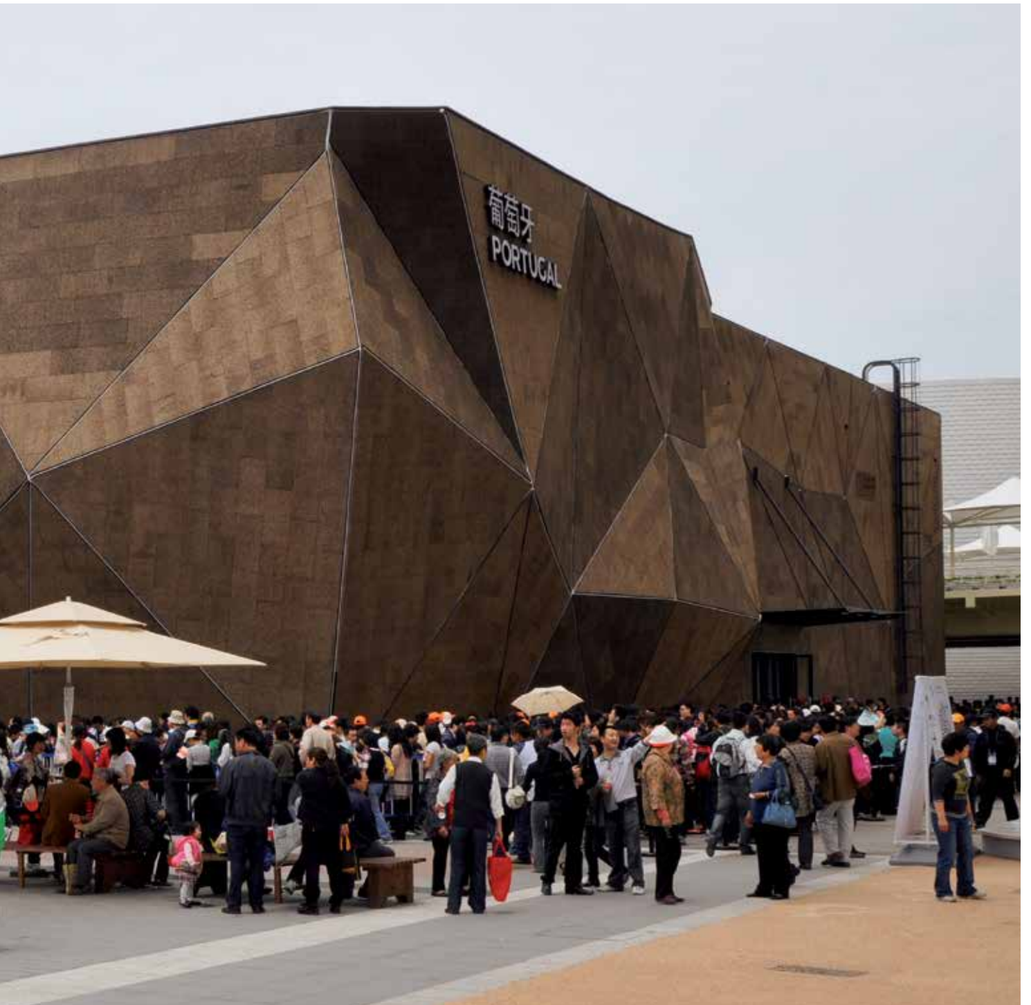
Portugal Pavilion in Shanghai (2010) with MD Façade
