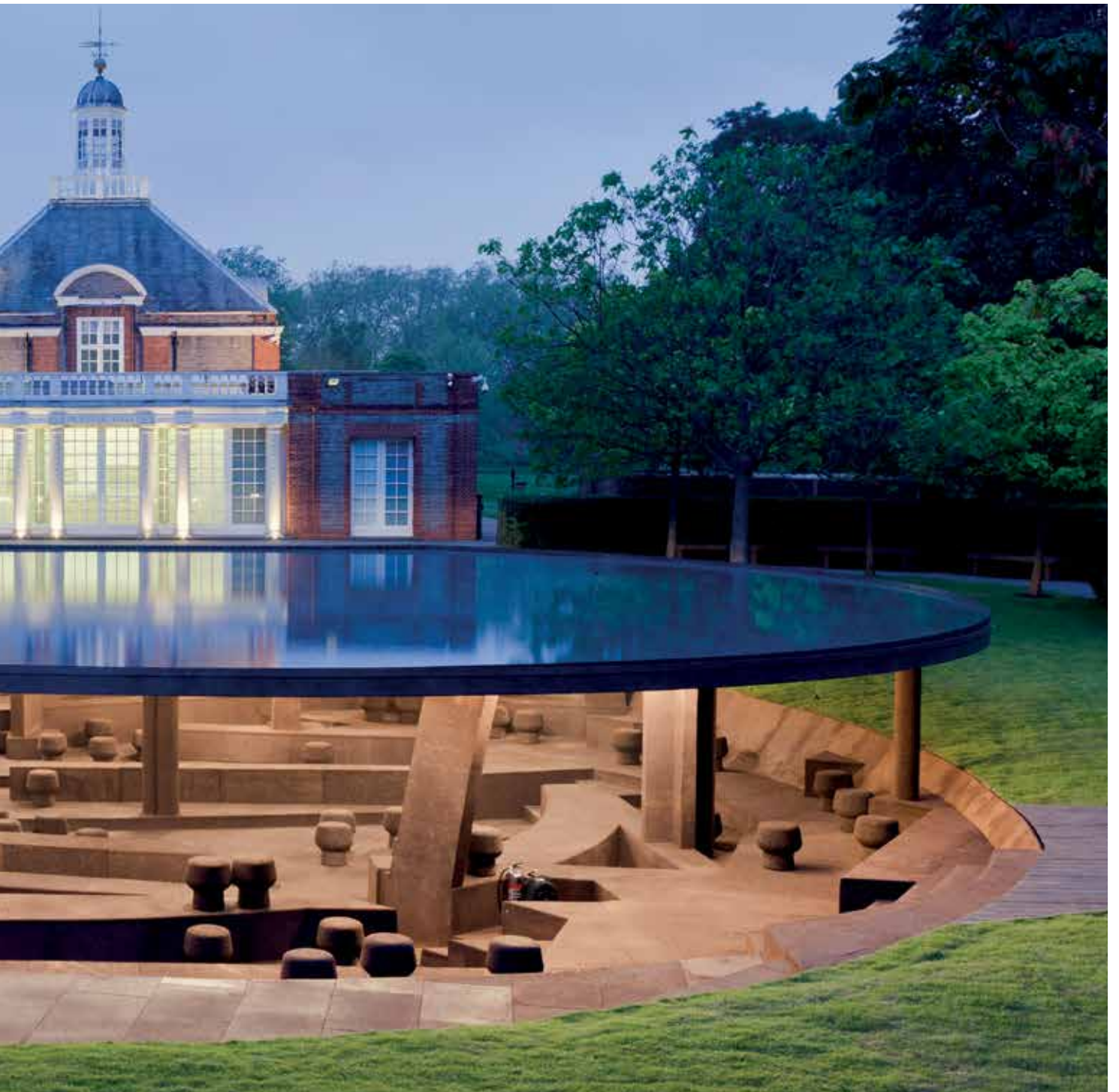
Serpentine Gallery Pavilion 2012, designed by Herzog & de Meuron and Ai Weiwei, with Amorim cork.
