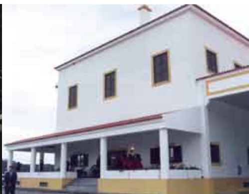
Façade of the new Drying Unit
