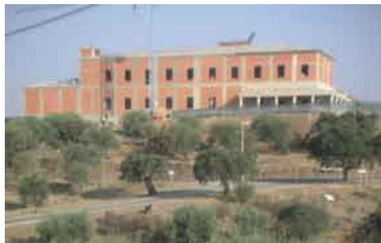
The new drying cell of Casa do Porco Preto will soon enter the finishing stages
